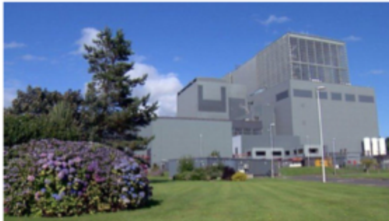
The total number of cracks found at Hunterston B's reactor three has risen sharply
