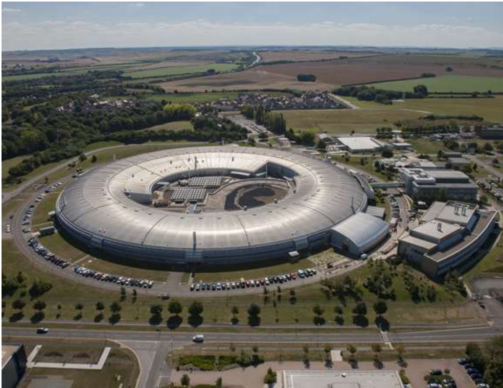
Figure 2. Diamond Light Source including Research Complex (RCaH), Diamond House (DH) & I14
