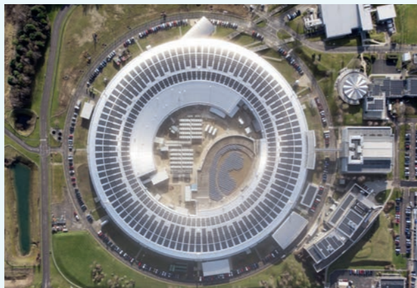
Figure 4. 2.7 MWp of solar panels installed on the synchrotron building roof.
