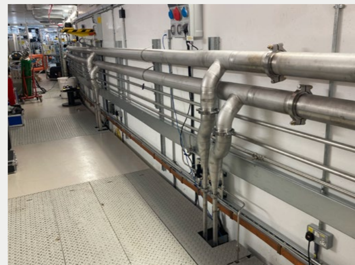
Demineralised A pipework upgrades
