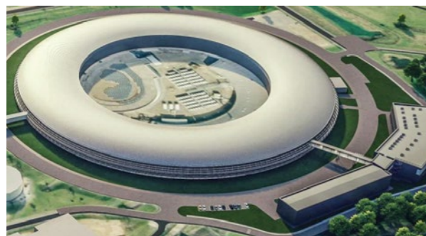
Architect's impression of the Diamond Extension Building (DEB), bottom right, to be constructed as part of the Diamond-II project, and link bridge to the synchrotron.
